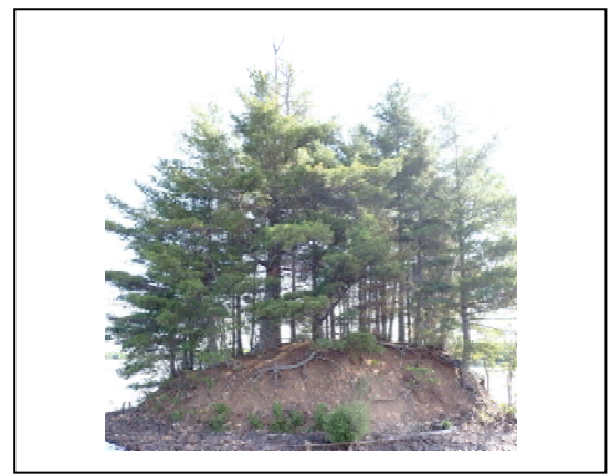
40. Island #8 – Bank erosion
