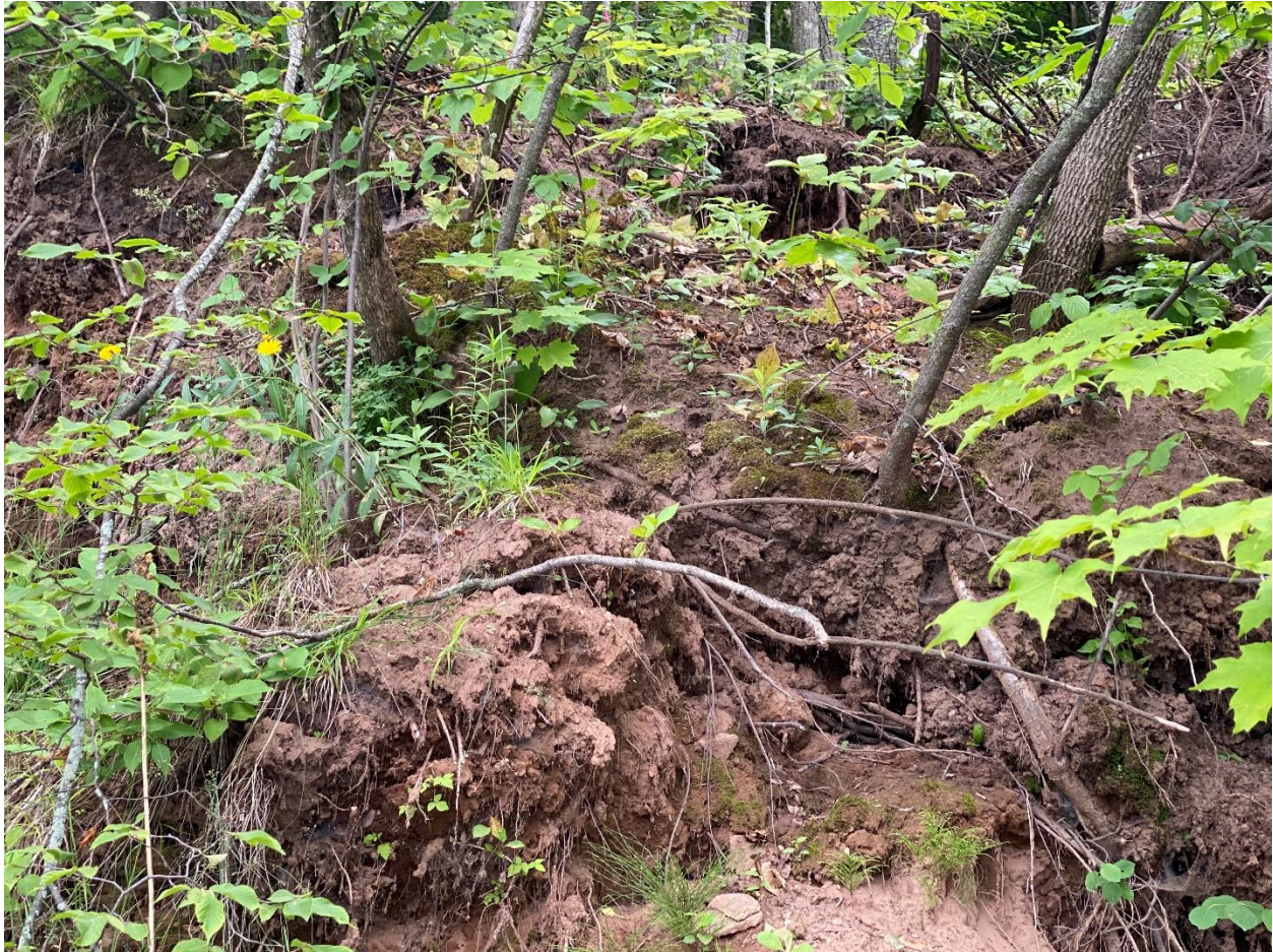
FIGURE 4g. SITE #5 GILE FLOWAGE (July 17, 2023). CLOSEUP PHOTOGRAPH OF BANK INSTABILITY
