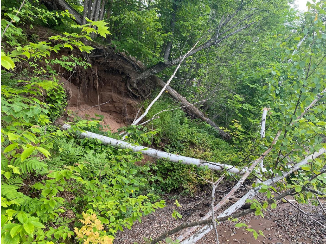
FIGURE 4d. SITE #5 GILE FLOWAGE (July 17, 2023). CLOSEUP PHOTOGRAPH OF BANK INSTABILITY
