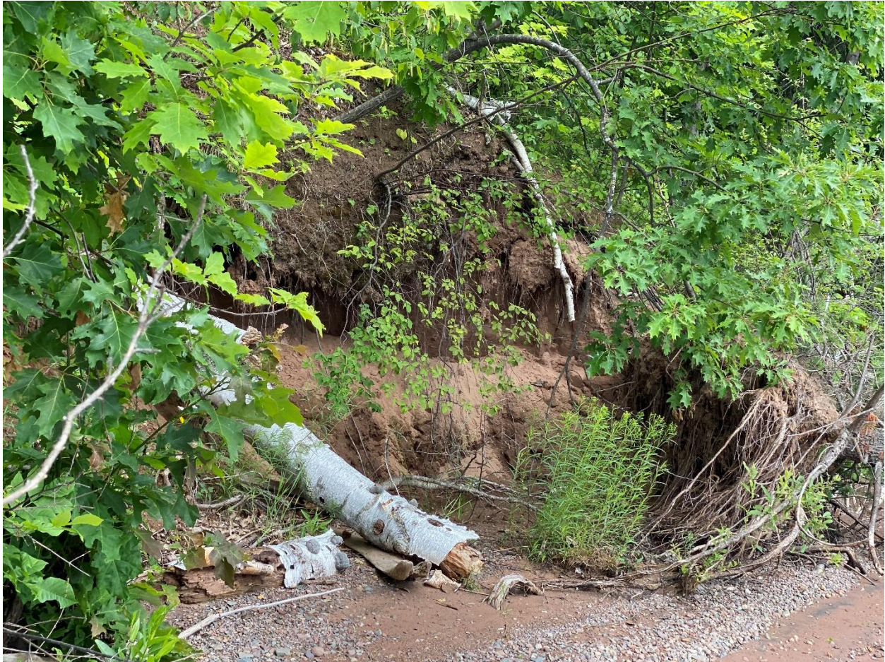
FIGURE 4i. SITE #5 GILE FLOWAGE (July 17, 2023). CLOSEUP PHOTOGRAPH OF BANK INSTABILITY
