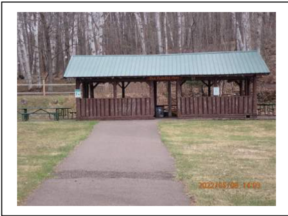
15. Gile Park – Pavilion and paved path
