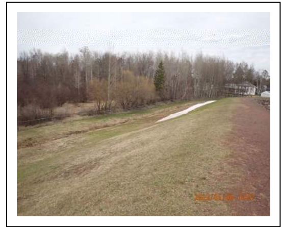
48. Gile Dam Canoe Portage – Dike walkway facing east
