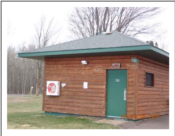
20. Gile Park – Restrooms (1)
